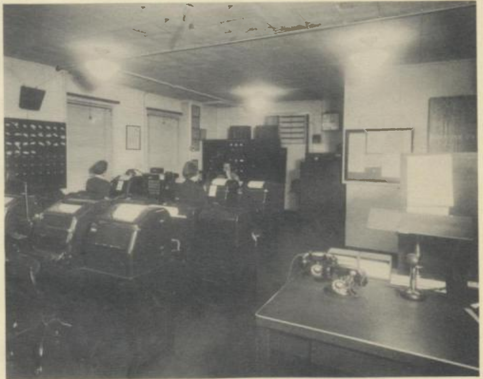
Teletype and radio equipment in the department's communications division at Hartford headquarters controls police teletype system of the state and the eleven frequency modulated radio stations of the State Police Department. Officer Frank R. Foley is shown at the radio control desk and Mrs. Grace McCann and Mrs. Katherine Allen at the teletype switchboard.
