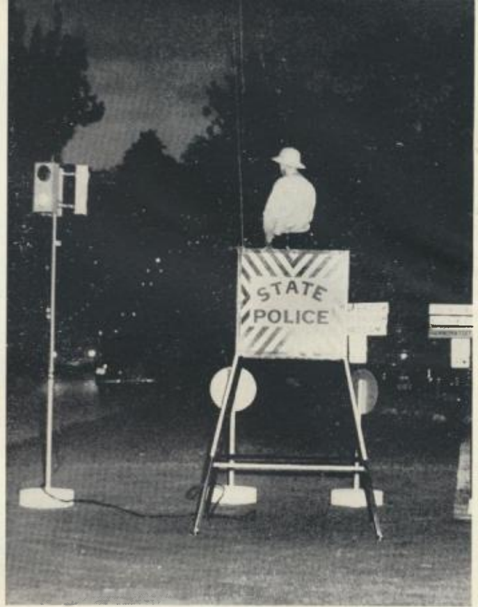
The portable traffic tower and portable signal lights shown above are used at points of heavy traffic congestion, such as shore points on Sundays in summer.
