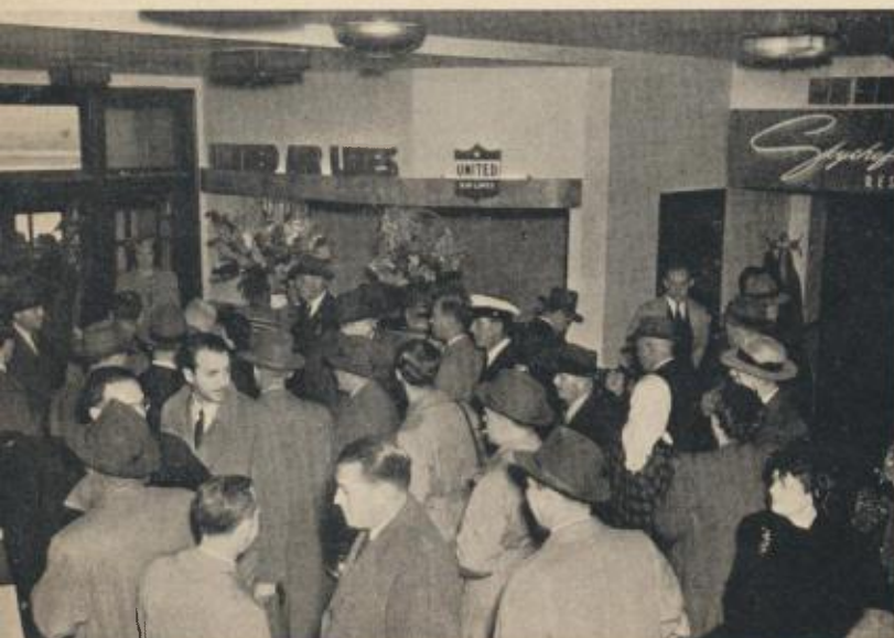
A part of the crowd which awaited the arrival of the first direct airlines flight from the West in the Administration Building at Brainard Field.
