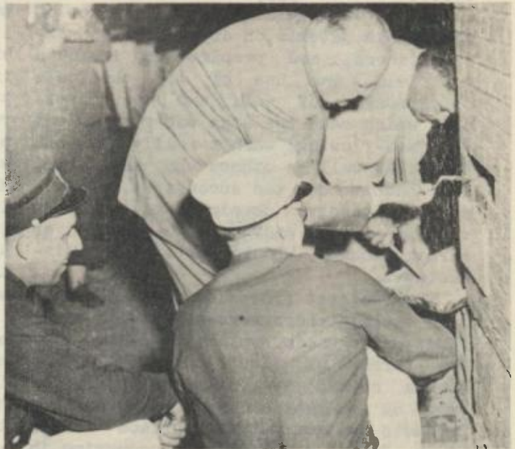
Police Comr. Edward J. Hickey is shown sealing the cornerstone of the new firehouse at Kent. At his left is First Selectman Theodore P. Woolin. In the foreground are Joseph Gawel, chairman of the building committee and Clifford Gustafson, fire chief.
